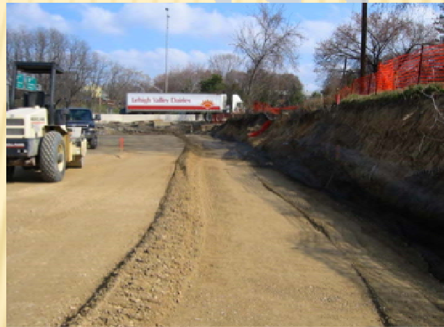
Placement of select fill for CSE from FHWA (2004).
