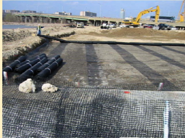
Placement of geosynthetic reinforcement for column supported embankment (CSE) from FHWA (2004).
